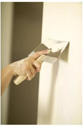
Repairing a wall using homemade materials is possible when the hole is small, the damage is minimal and the wall is constructed of drywall. Stucco, plaster and panel walls are not easily repaired, and even less so using materials lying around the house. If you have a few small holes or dings in a drywall wall, there are a few ways to repair them and prepare the area for a coat of paint.
