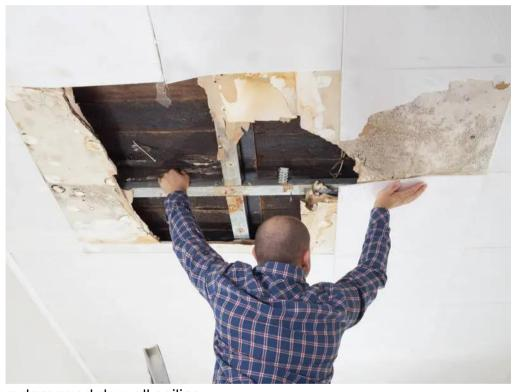
To repair a damaged drywall ceiling:
